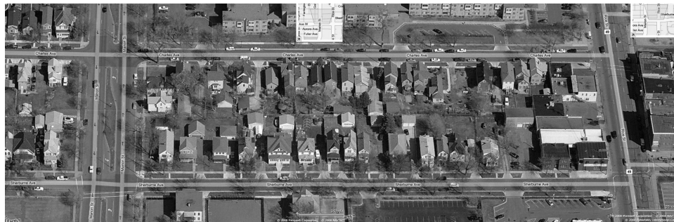
Examples of Typical Buildings and Views, RM District
